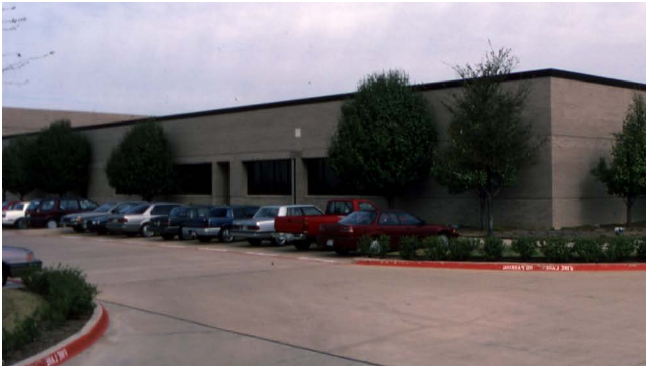
GTE SALES AND SERVICE CENTER Irving, Texas
